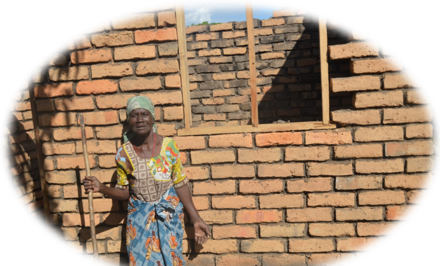
Eluby Semeon standing in front of her house which is under construction
