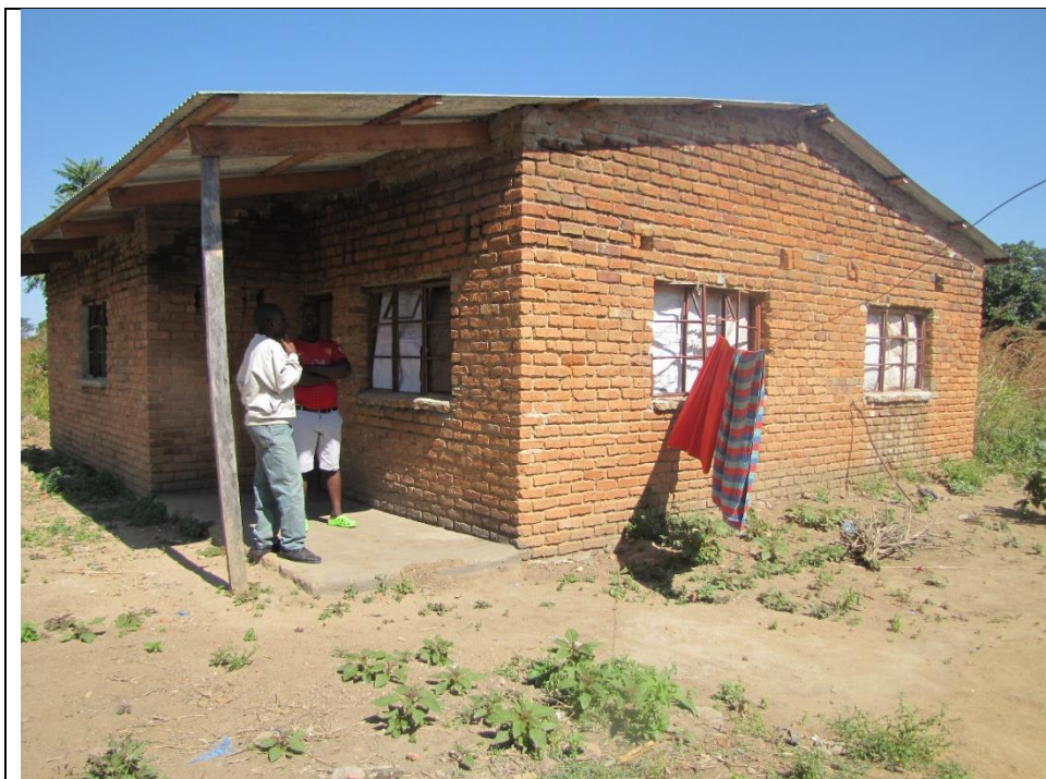
A house for a Police Officer at Katowo in Rumph West Constituency, though incomplete benefited from CDF funds in 2016/2017
