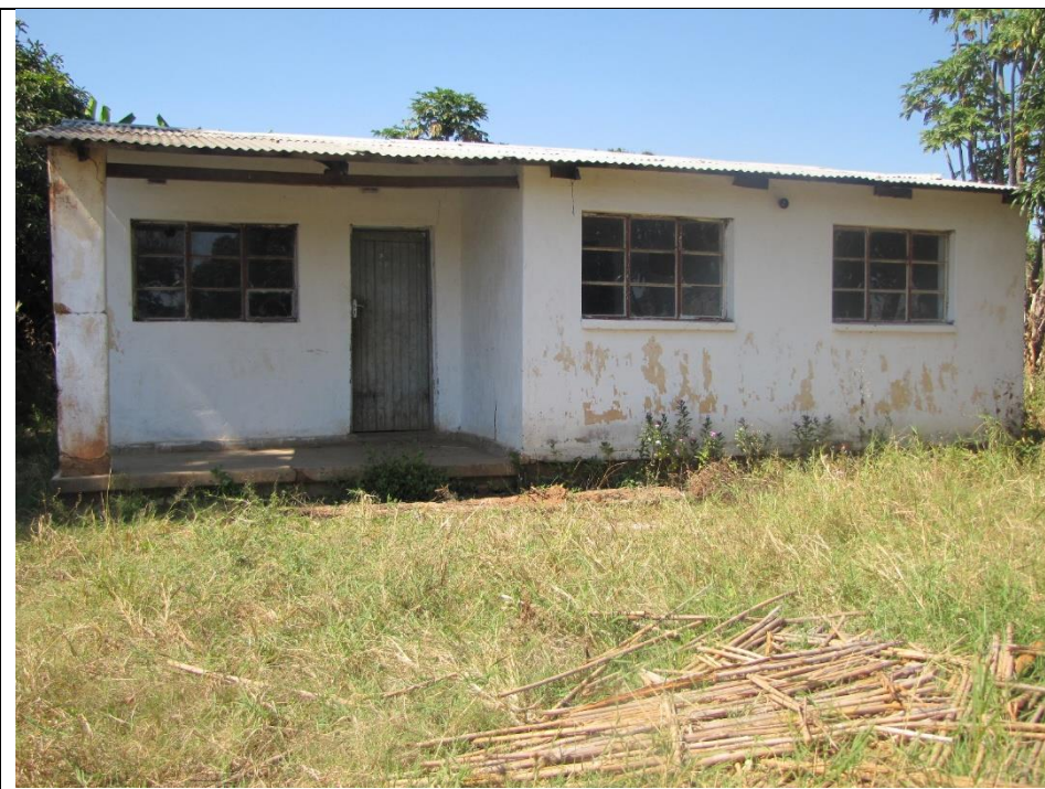
A CDA's house at Katowo, in Rumph West Constituency that benefited from CDF Funds in 2016/17 fiscal year. Wiring for electricity was done.
