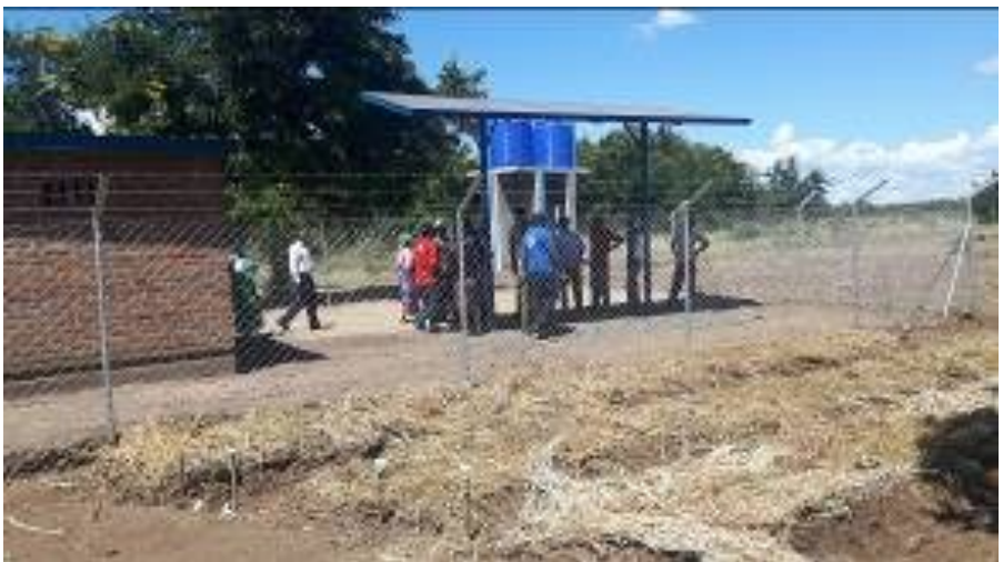
Stakeholders appreciating the solar panel which is expected to provide the much-needed energy to the hydrants.
